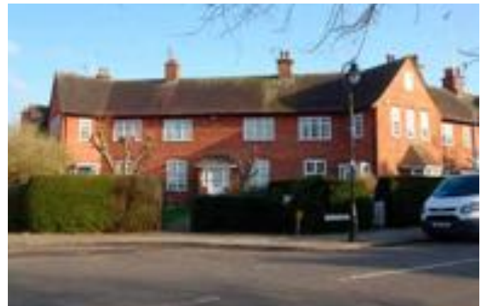
Corner terrace at Brentham Garden Suburb, Pitshanger
