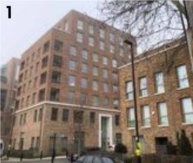
1 Acton Gardens perimeter blocks and town houses
