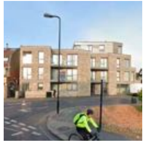
Modern block of flats
