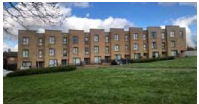
Goshawl Court: a terrace of townhouses, on sloping land in Sudbury Hill
