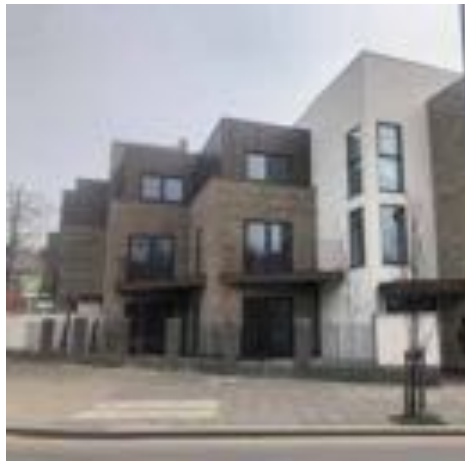
Modern block of flats
