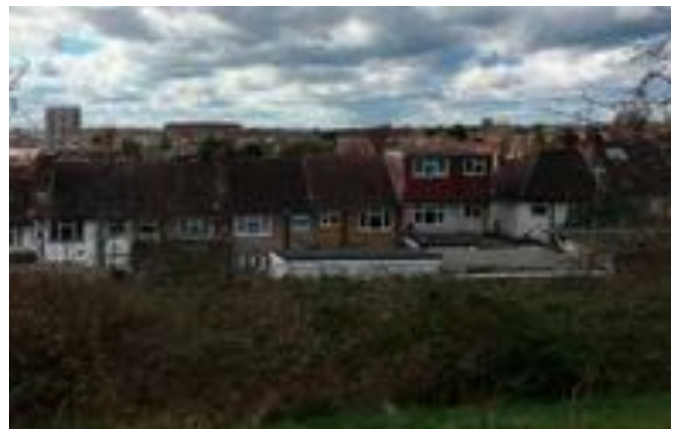
Views southwards from Sudbury Hill towards Greenford Quays
