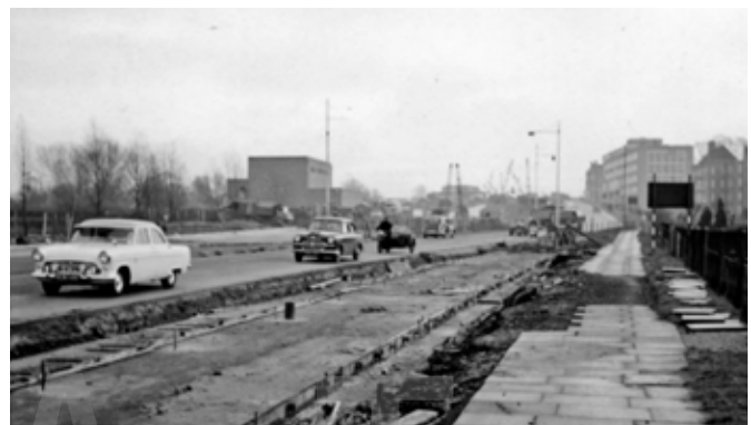
North Circular Road under construction in the 1930s
