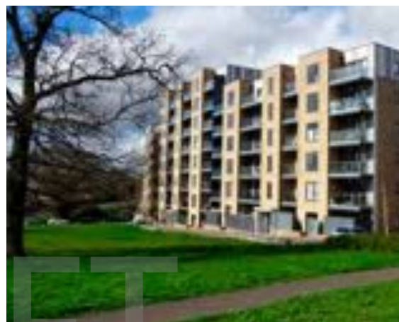
Goshawk Court, Subury Hill is a recent example of residential intensification that abuts railway lines and will have had to incorporate noise mitigation measures.
