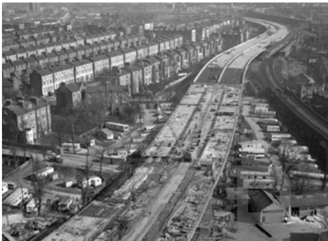
Construction of the Westway in 1970
