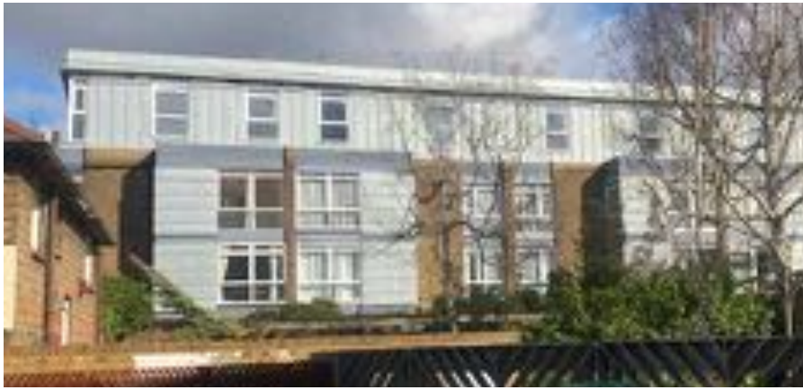
A residential block with a single storey extension in west Ealing
